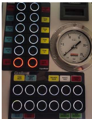
Example Fire Panel switching/level lights with LED indication
